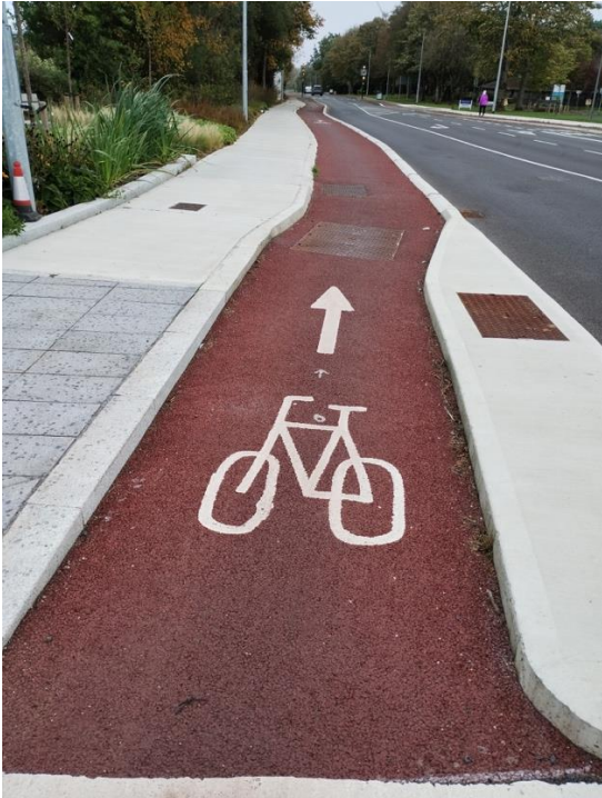
Fig 1. Plassey Park Road: recently constructed cycleway.
