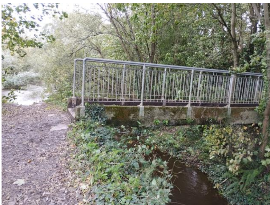
Fig 3 The recently repaired footbridge over the ditch.
